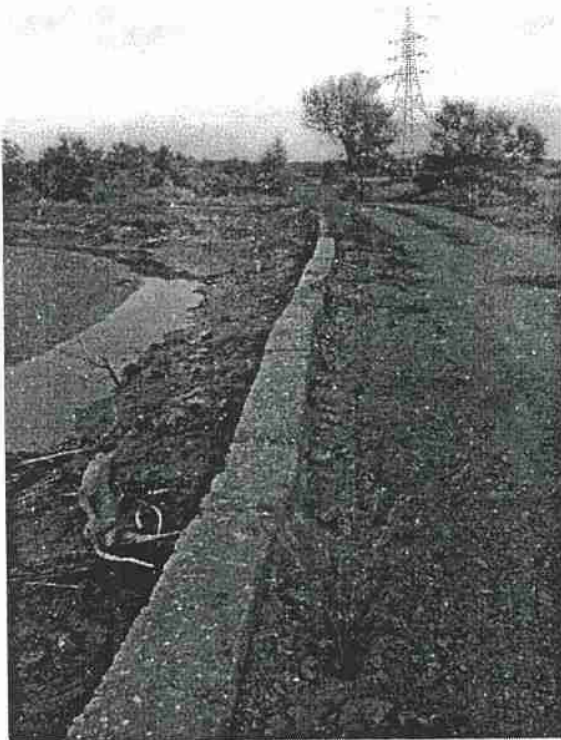
Left: Northern part of the embankment closer to the river; the wall all along the outer periphery of Cavso Cantor bundh is already built some years back. Right: The trench is dug for the foundation of the proposed works; the original embankment is completely buried by red mud.
